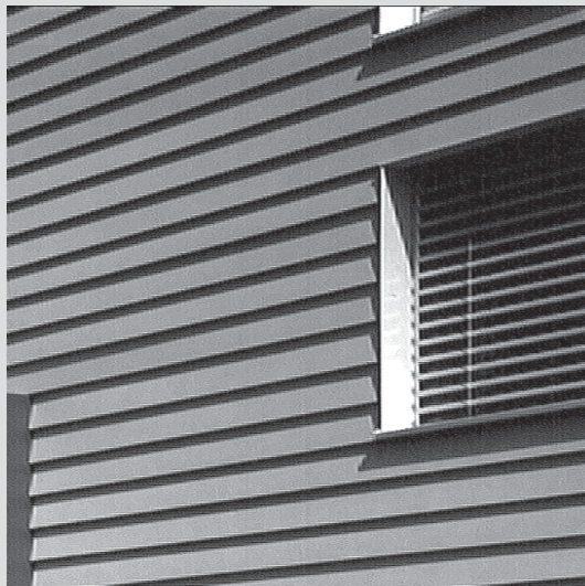
Planks with spacers to emphasise the laps
