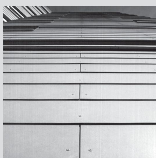
Tight lapped panels, staggered joints, color matched rivets
