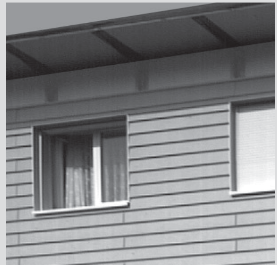
Tight lapped planks, staggered joints, concealed fixing
